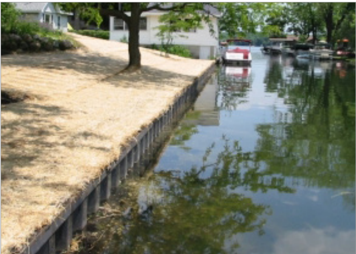
Shoreline Enhancement Option - Sheet Piling
