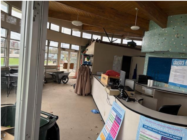
Entrance at pool cashier desk looking south. Spheroidal glass lights above.
