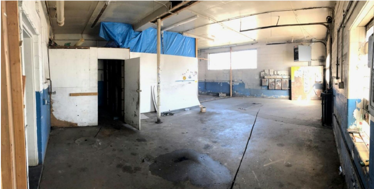
Back Bay Area #2 and supply closet
