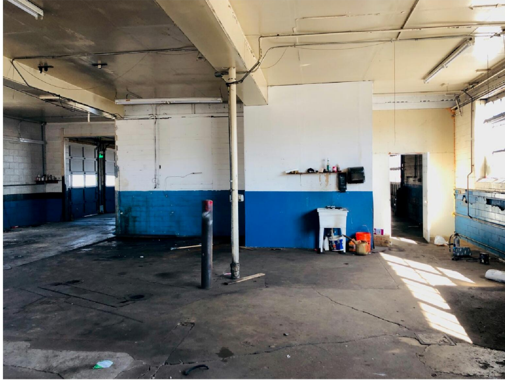
Repair Bay Area #2- East side of building
